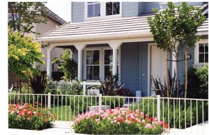
Porches are a dominant feature at streetscape
